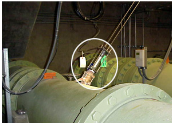
The Multi-Mag (highlighted above) is ideal for applications where space and straight pipe runs are at a premium.
