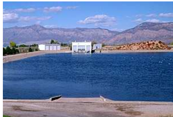
Pumping house on on of the system's resevoirs.
