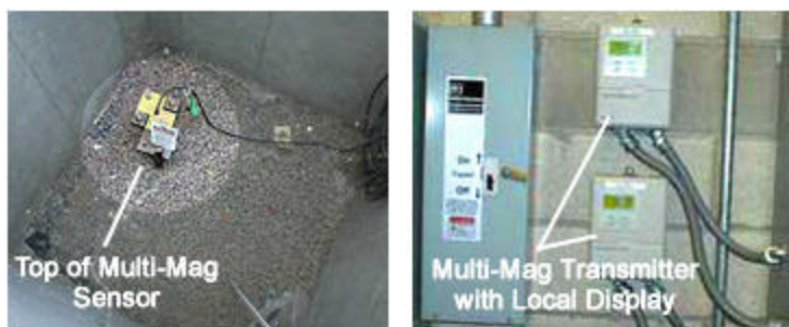
One of West Kern's Multi-Mag Sensors (left) and two of their transmitters (right).
