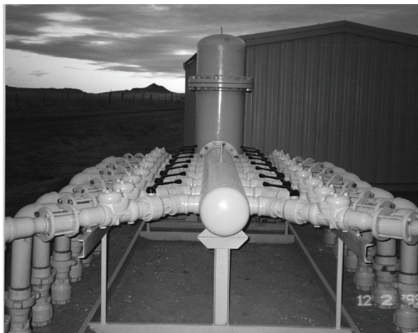
Figure 6. Pod system Wafer-Cone (16 units in same envelope as 7 orifice)
