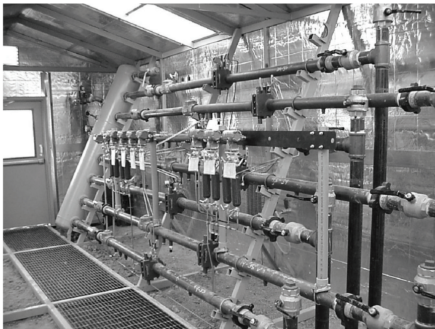
Figure 5. Pod building design using orifice meters (envelope for 7 units)
