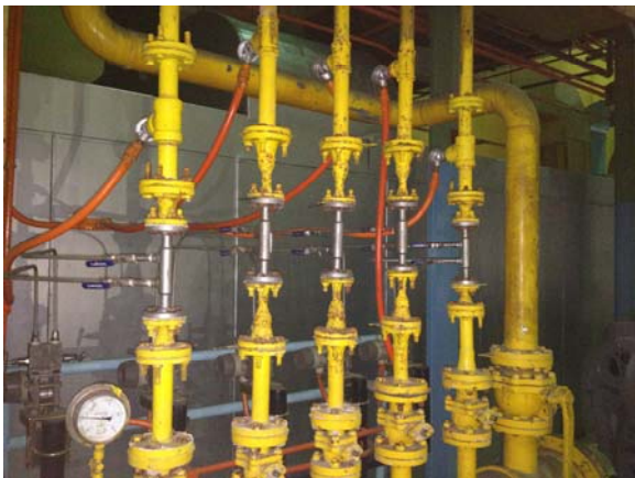
Figure 1: V-Cone Flow Meters Installed In A LPG Piping Application
