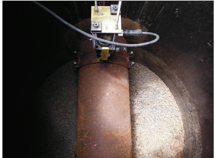
The FPI Mag flow meter installed at the caprock well
