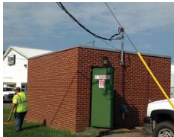
Figure 1: Buckhannon's Tennerton Booster Station
