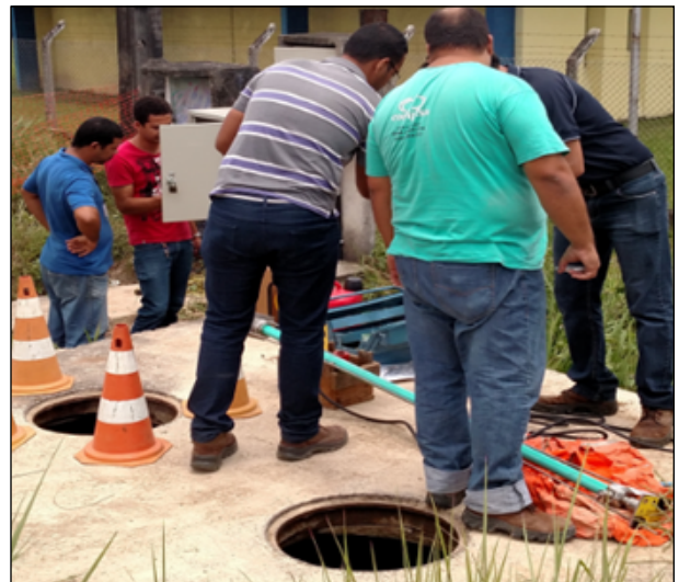
Preparation for FPI Mag meter installation
